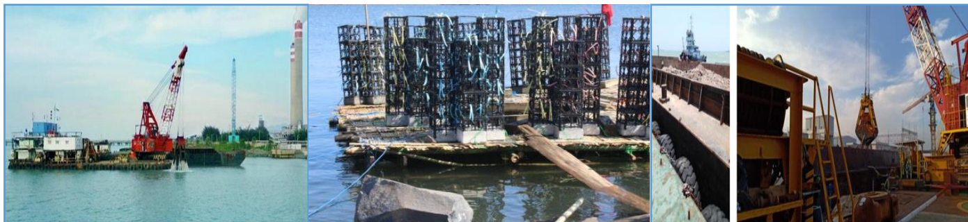
FIG. 1. a: Fish apartment; b: Grabdredger dredging activities; c: Transport of bottom type hopper barge.
