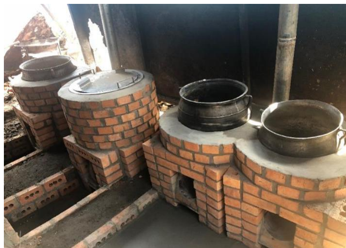
FIG. 3. A completed set of institutional cook-stoves. Here we have round and flat bottoms
